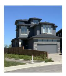
The upper storey must be set back a minimum of 2' from the middle storey with a roofline bridging the 2 floors (with limited exceptions).
